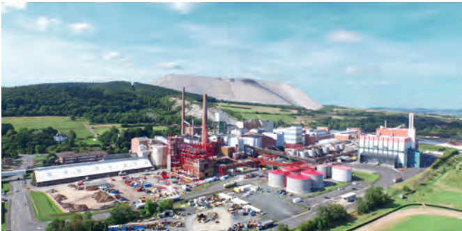
Werra 2060: restructuring potash production plant – Germany Owner's engineer and advisory services for the restructuring of the plant to modernize processes, reduce CO 2 emissions, improve water management, and enhance sustainability
