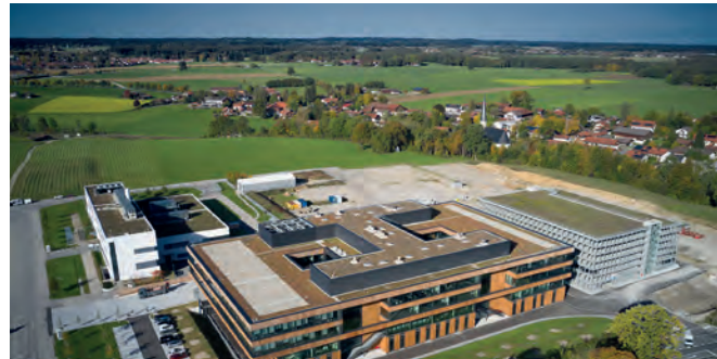
Bosch, HK0202 new development center – Germany Plumbing, air handling, energy, sprinklers, building management systems
