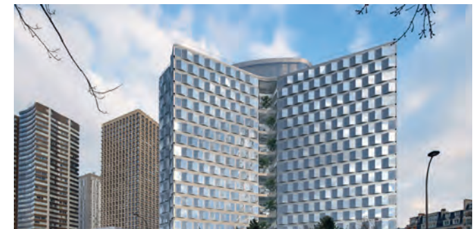
Mirabeau Tower Rehabilitation – Paris, France Technical studies and design, construction supervision
