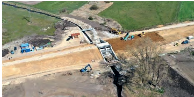
Donauwörth retention basin – Germany Execution, assistance for the awarding of contracts, safety, health and protection coordination
