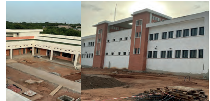
Teacher's Schools – Bouaké & San Pedro, Ivory Coast Design and construction supervision
