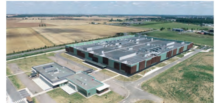
Orange data centres – France Design and construction supervision
