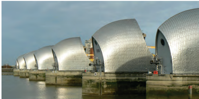
Thames Barrier – London, United Kingdom Engineering design, tendering and construction supervision
