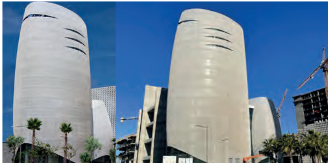
Construction of CIMR Headquarters – Casablanca, Morocco Project Management
