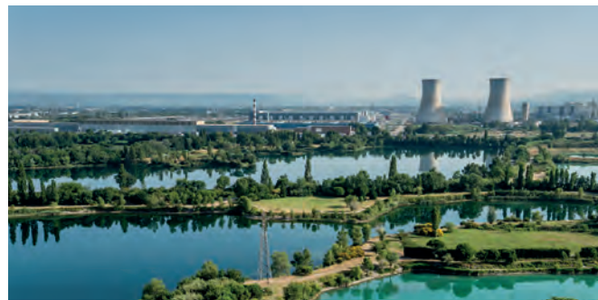
Orano Pastel project: facility for treating uranium effluent – France Expertise in nuclear processes: analysis of various evaporation technologies, sizing, energy efficiency optimisation and safety assessment for filtration technologies
