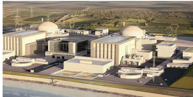
Hinkley point C turbine hall – United Kingdom Detailed civil engineering design for nuclear island buildings
