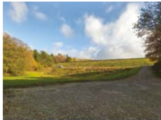
Saint Pardoux Dam
