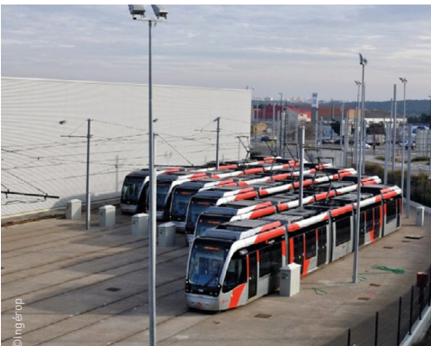
© Ingénierap ZARAGOZA TRAM (SPAIN)
